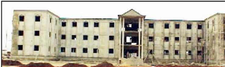
Main Campus The gigantic structure awaiting final touches
